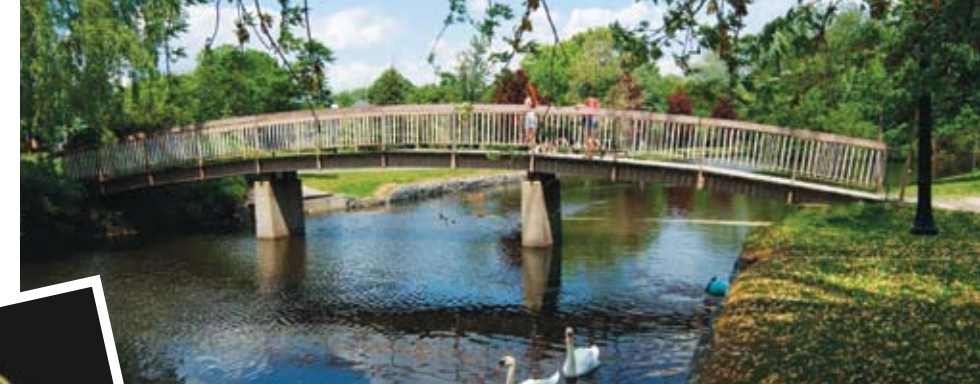
Bridge at Victoria Park.
